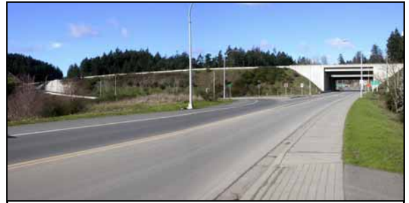
Figure 4 Recently Constructed Fill Slope
