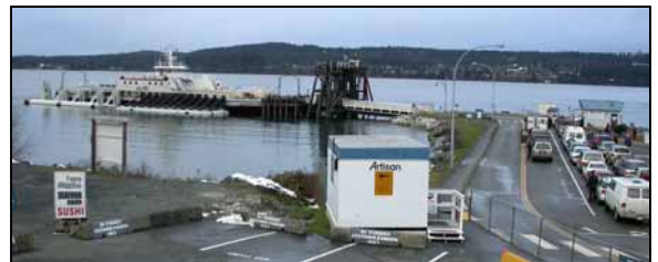
Figure 6 Ferry Terminal Marine Structures
