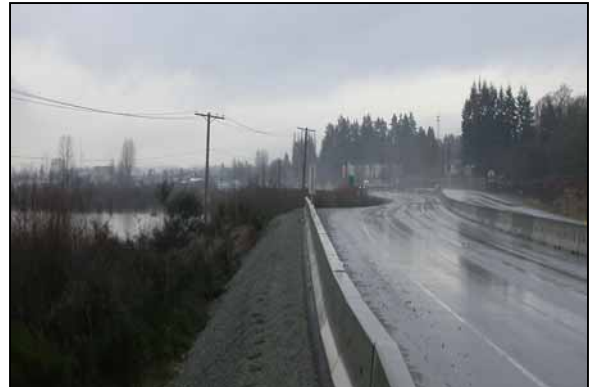
Figure 5 Fill Potentially Subject to Liquefaction
