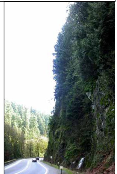
Figure 3 Potential Rockfall Hazard
