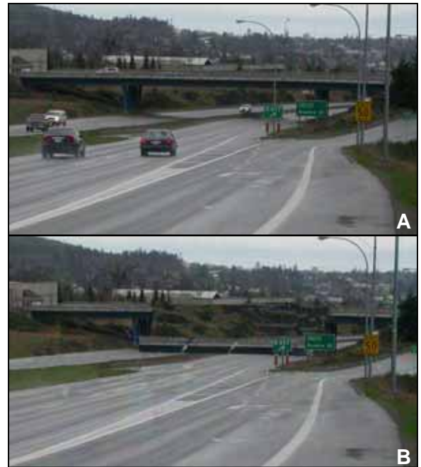
Figure 1 Potential Bridge Failure
