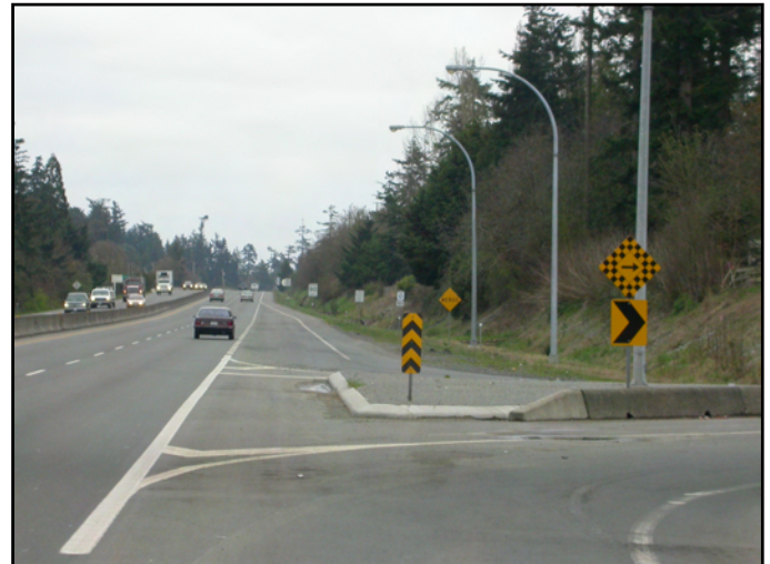
Figure 4 Exit gore signs
