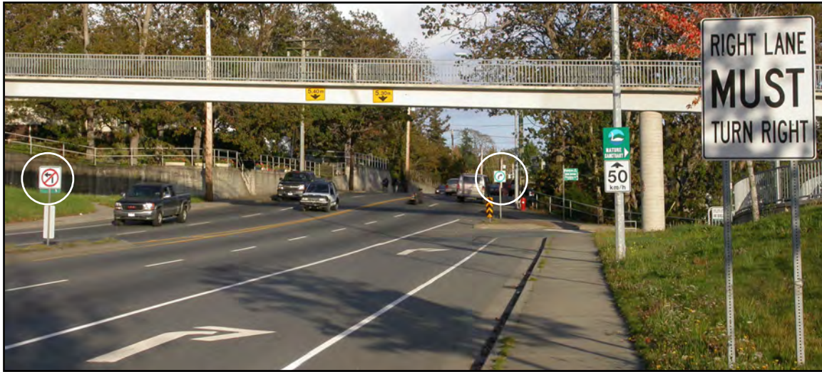
Figure 5 Incorrect combination/use of Turn Control signs (median and far end of right lane)
